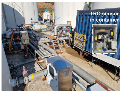
(a) Ballast water treatment facility
